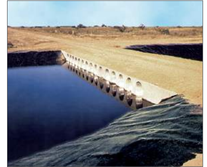
GSE lined canal with incorporated flow control system
