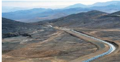
[GSE lined canals help prevent water loss]
