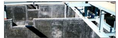
[GSE Liner in wastewater treatment aerobic digester]
