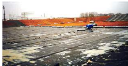
[GSE GundSeal in a food processing Sludge Lagoon]
