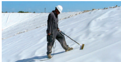
[GSE Leak Location Spark Testing]
