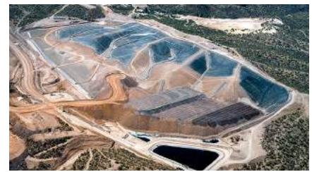
[Mine Drainage Operation]
