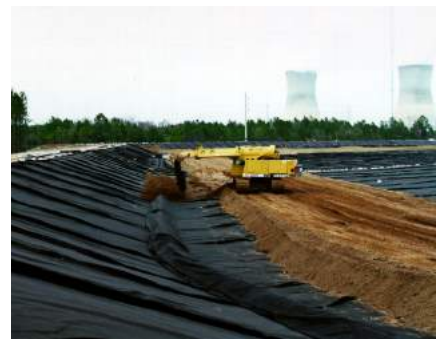
[Cooling Water Pond Storage]
