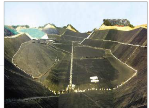
LANDFILL WASTE PIT
