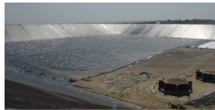
[Hydro Power Plant Application]
